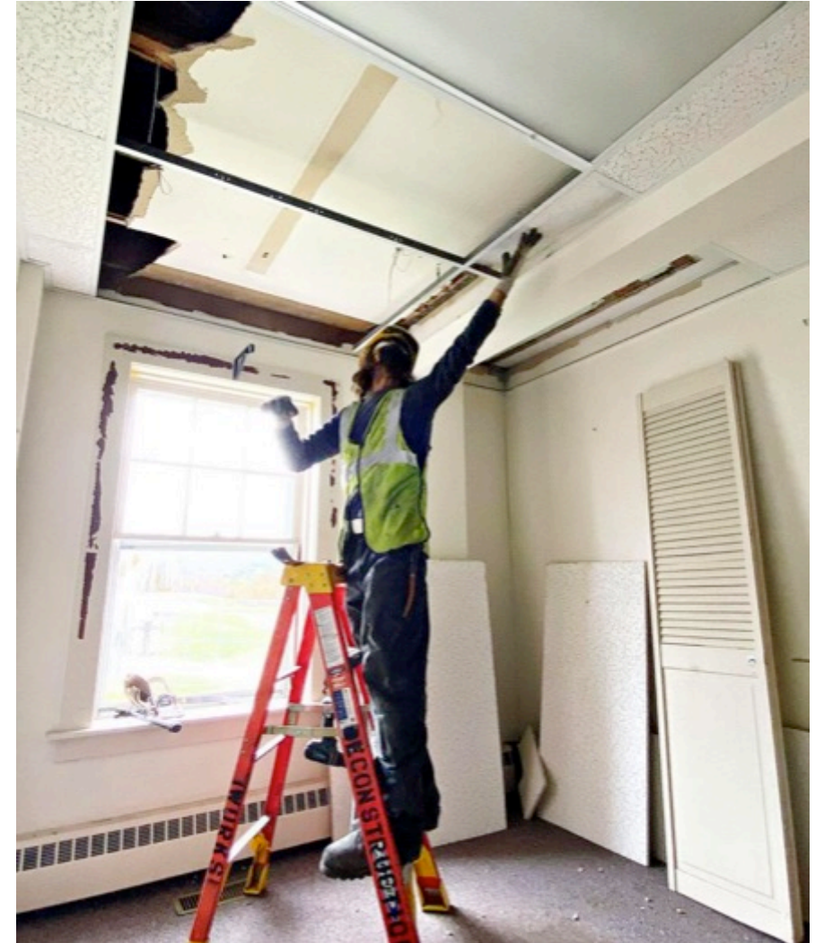
SOURCE: BENNER HOSPITAL DECONSTRUCTION
